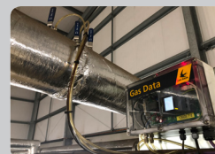
Gas Flow Monitoring
